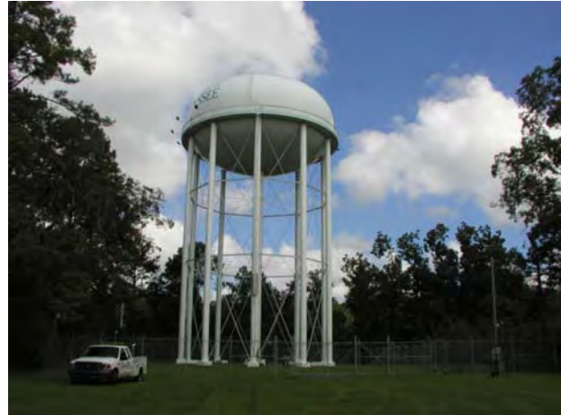
Example No.2 – Elevated Storage Tank (600,000 gallon capacity)
