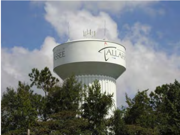
Example No. 1 – Elevated Storage Tank (1,000,000 gallon capacity)
